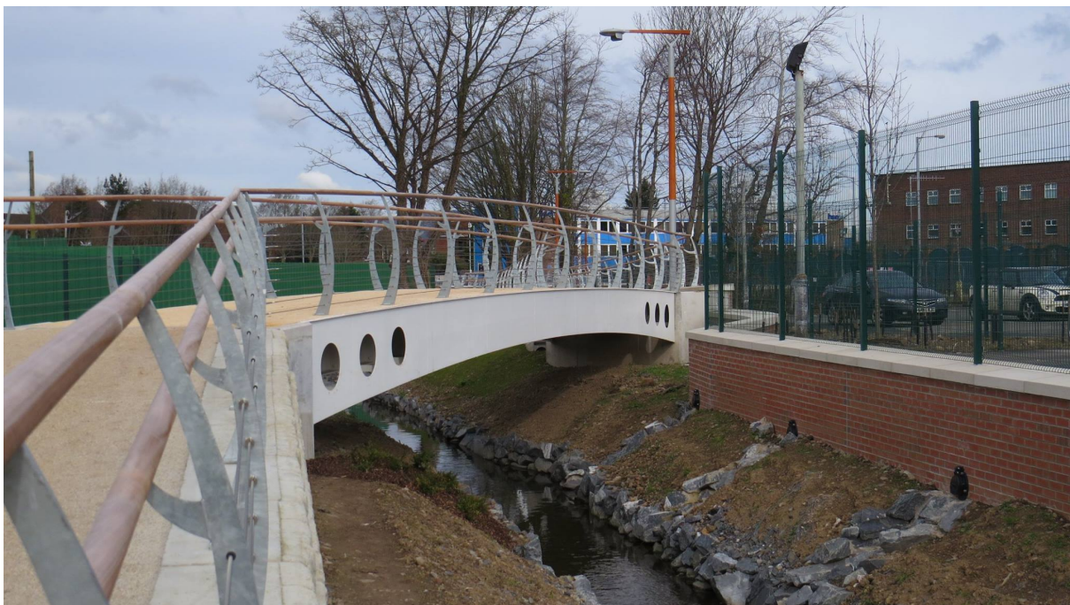
Bridge at Alexander Road
